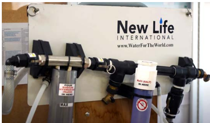
Figure 2: NLI's water purification system makes water safer for people in developing countries around the world. The purifier can treat up to 55 gallons per minute and produces water that is free from harmful bacteria.
