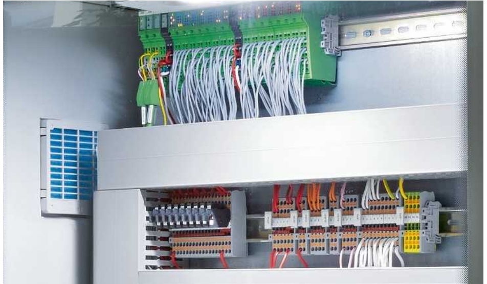
Fig. 11: Front connection technology with cable outlet on one side and conductor outlet on both sides in the cable ducts
