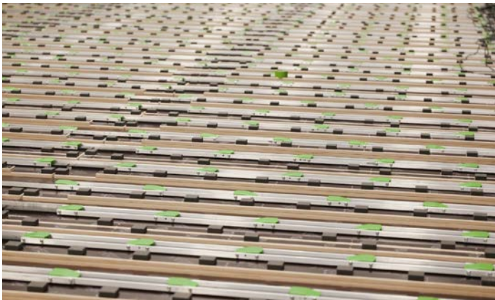
Figure 2: The mechanics beneath the floor make it easy to switch between a sprung and rigid surface.
