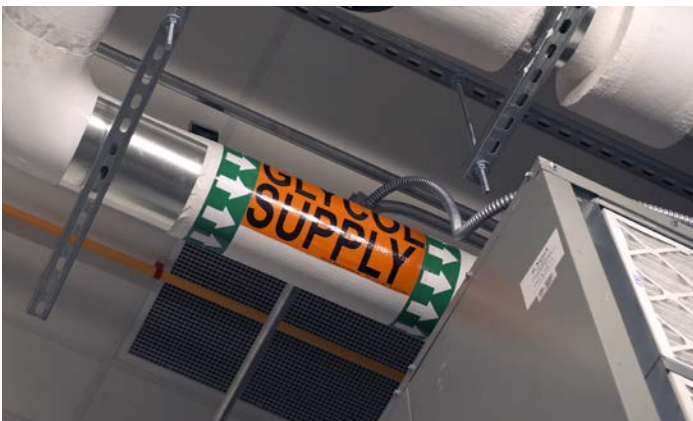
Figure 2: NOVVA uses a glycol mixture, rather than water, to keep its data centers cool.
