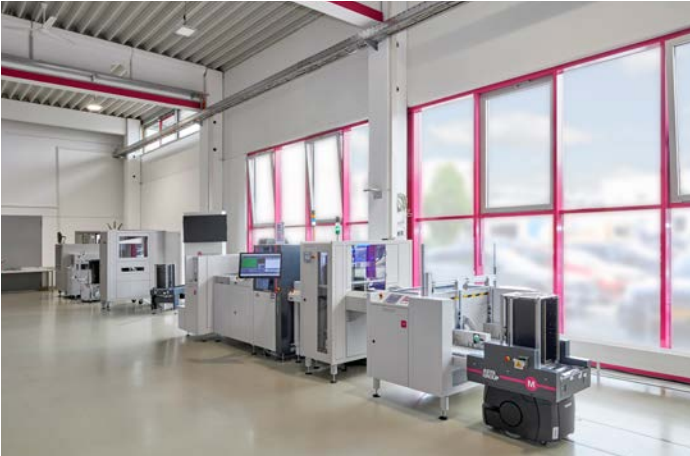
Figure 2: The Pulse assistance system is used to monitor individual line configurations.
