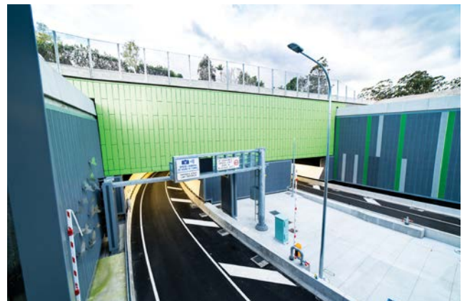
Figure 1: Sensitive adjustment of the lighting conditions to the increasing darkness in the tunnel is already necessary at the entry point. (Image source: Transurban/NorthConnex)
