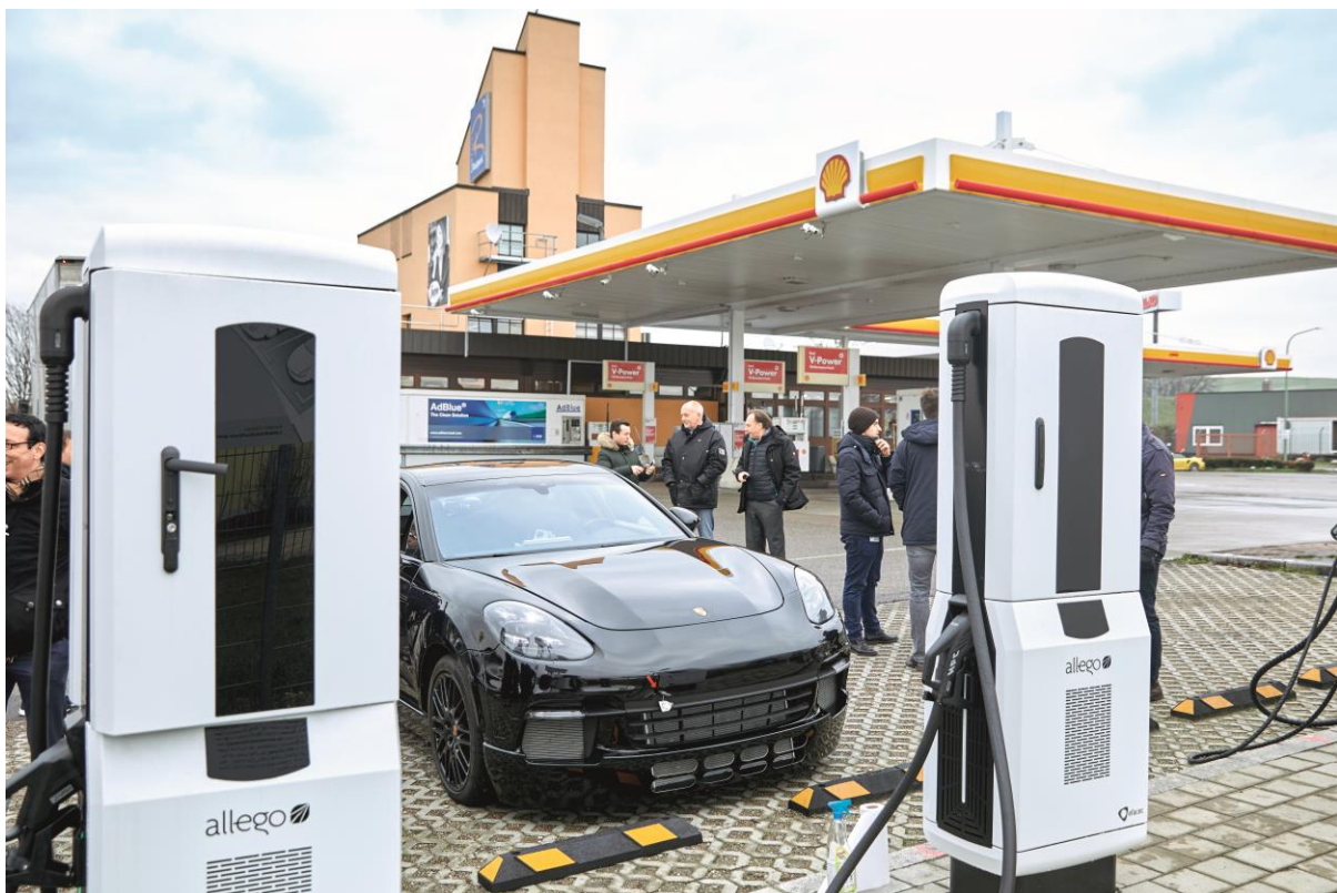
Figure 3 - New record: the charging station on the right provides 450 kW and the other one on the left charges at 175 kW
