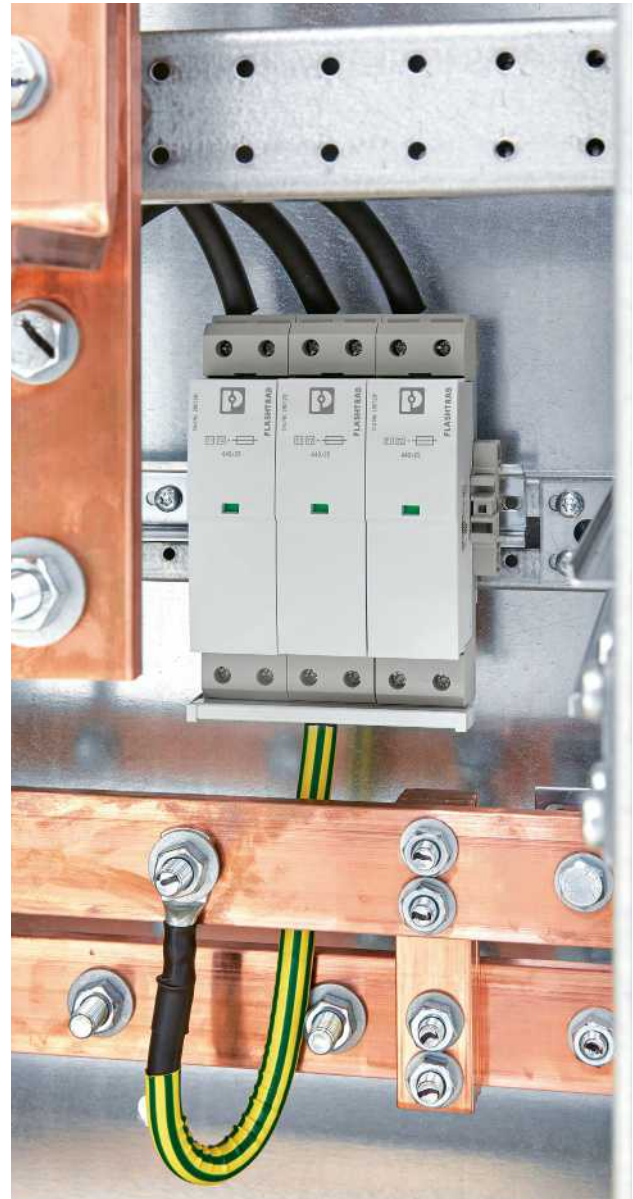
Type 1+2 combined lightning current and surge arrester with integrated fuse FLT-SEC-H-T1-3C-264/25-FM Order No. 2905871
