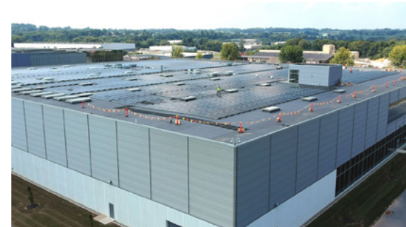
Solar panels generate nearly 1 MW of electricity at Phoenix Contact USA headquarters
