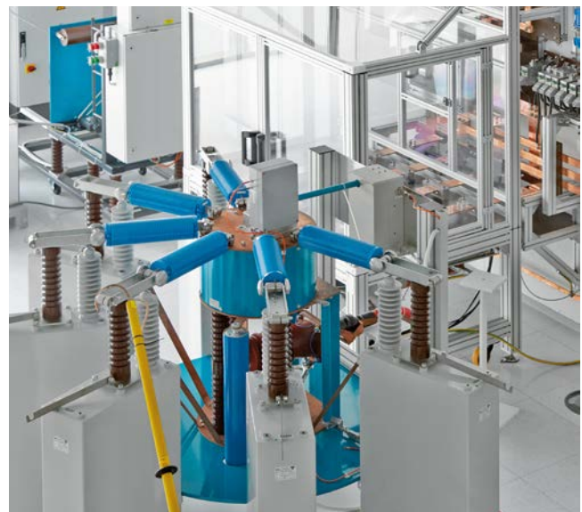
Figure 2: Components and devices from manufacturers being tested in the high-voltage lab
