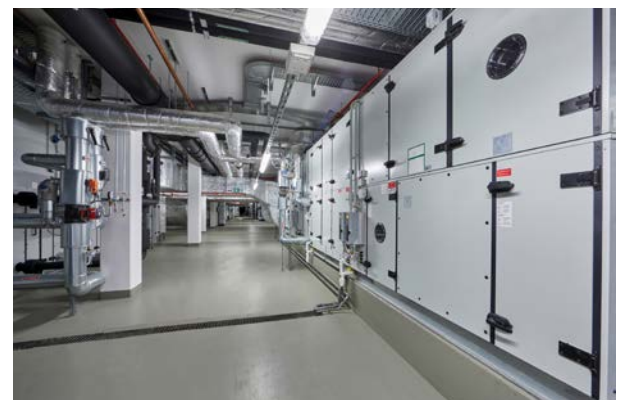
Figure 1: The switching devices were modernized in the first step.
