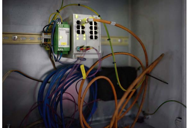
Figure 2: The managed switches from Phoenix Contact ensure a failsafe network with their redundancy mechanisms and numerous diagnostic functions.
