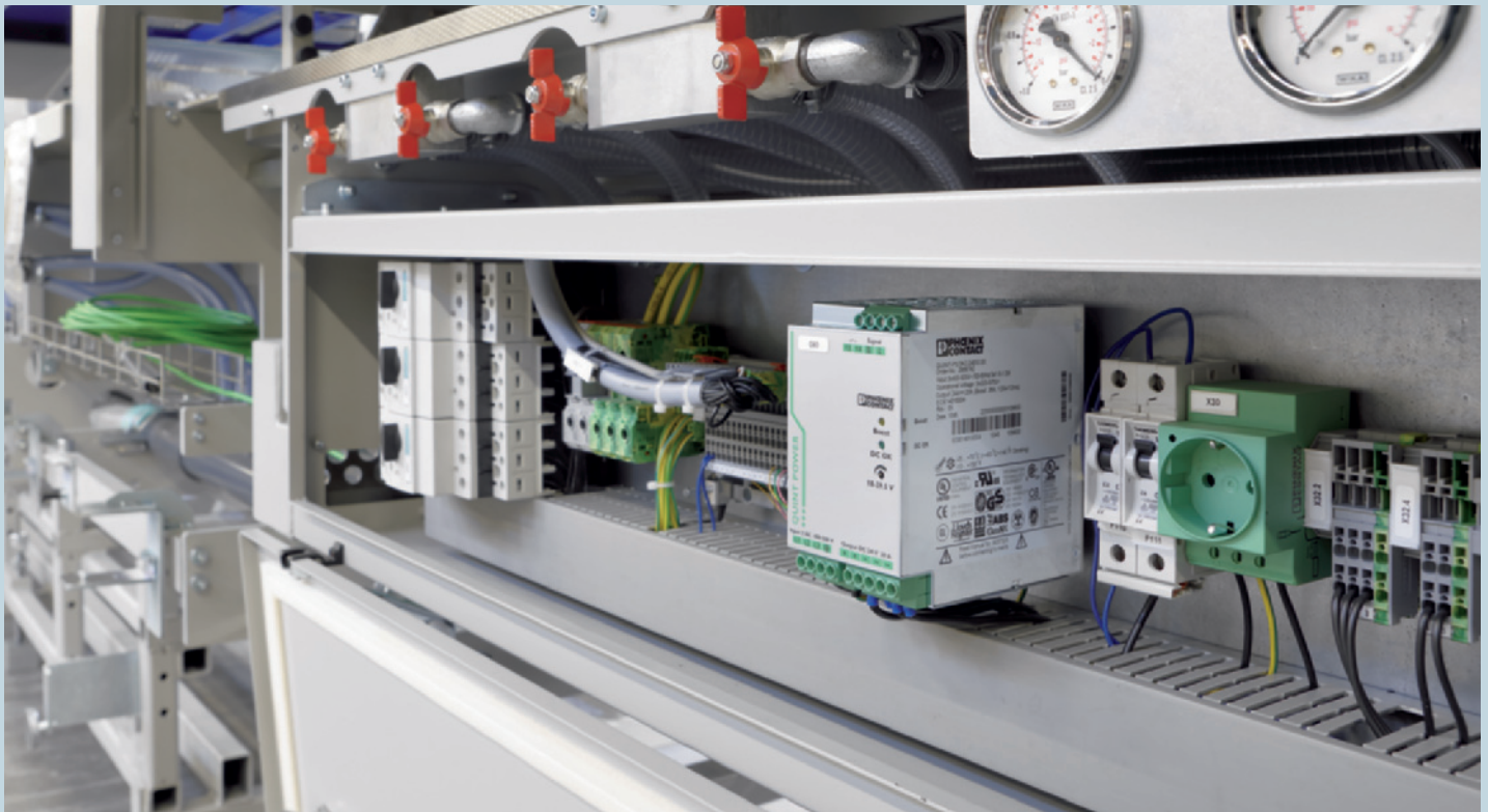
A power supply unit with SFB technology guarantees fast and safe tripping of device circuit breakers in the event of an error
