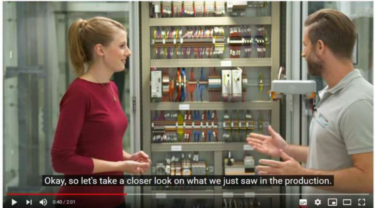
Network infrastructure for control cabinets with COMPLETE line
