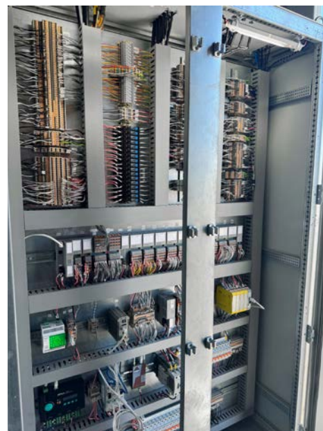
Figure 3: The control cabinet of the power bank systems is equipped with standard and safety controllers, surge protection, cables, terminal blocks, lighting, I/O systems, Ethernet switches, and communication gateways from Phoenix Contact. (Image source: Endua)
