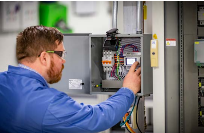
Figure 2: Basic energy meters, like the Phoenix Contact EMpro, can measure and collect system conditions like voltage, current, and power.
