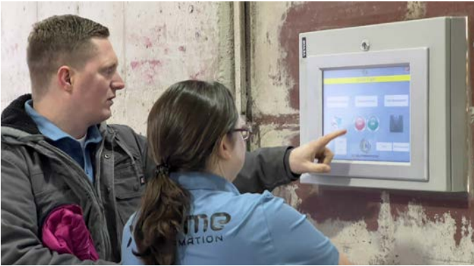
Figure 2: Operators use the touchscreen interface to select the grain's destination.
