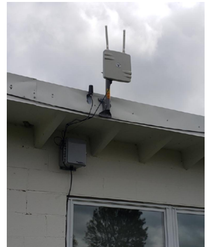
Figure 1: The FL EW-EW75000-08 radio provides IP67 outdoor wireless access points (WAP) with high-speed wireless connectivity for harsh and demanding environments.
