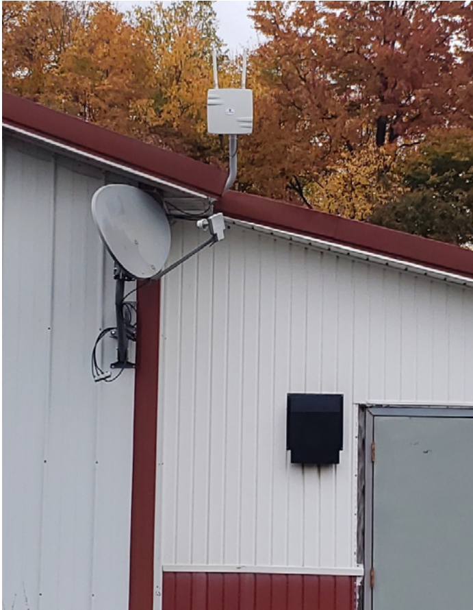
Figure 3: RAFA Systems installed nine access points around the district, including some rural locations.
