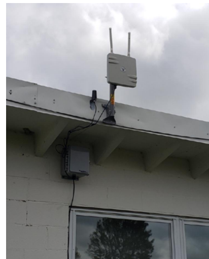
Figure 1: The FL EW-EW75000-08 radio provides IP67 outdoor wireless access points (WAP) with high-speed wireless connectivity for harsh and demanding environments.
