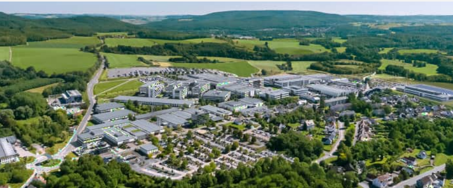
Headquarters Blomberg | Germany
