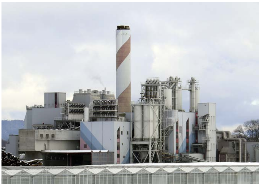
Industrial colossus with high-tech hood: filter system on the roof of the garbage incinerator
