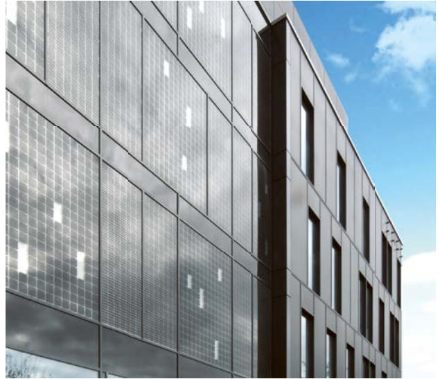
Innovation in detail – photovoltaic elements are integrated into the façade modules on the south side
