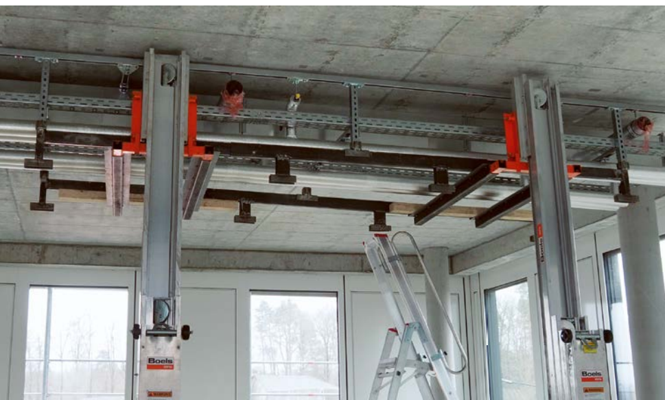
The pre-assembled TBU modules are installed in no time at all
