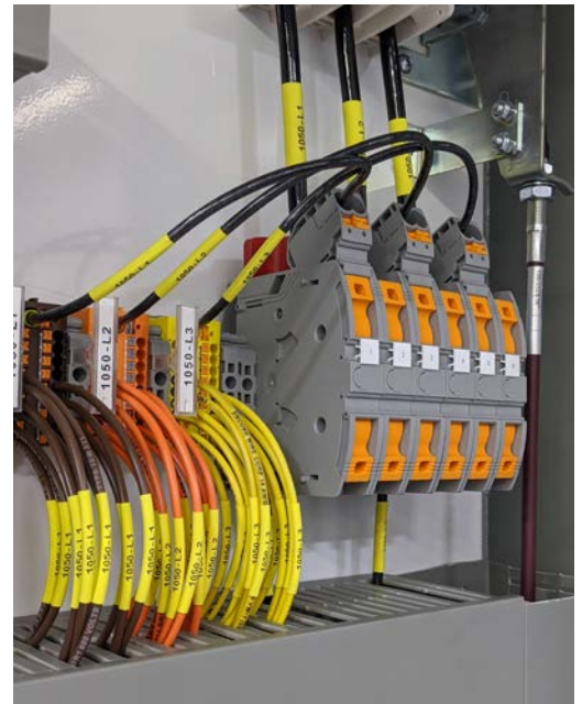
Figure 2: PTPOWER offers fast, user-friendly connection for wiring large conductors. Novum now uses PTPOWER for nearly all of its power distribution.
