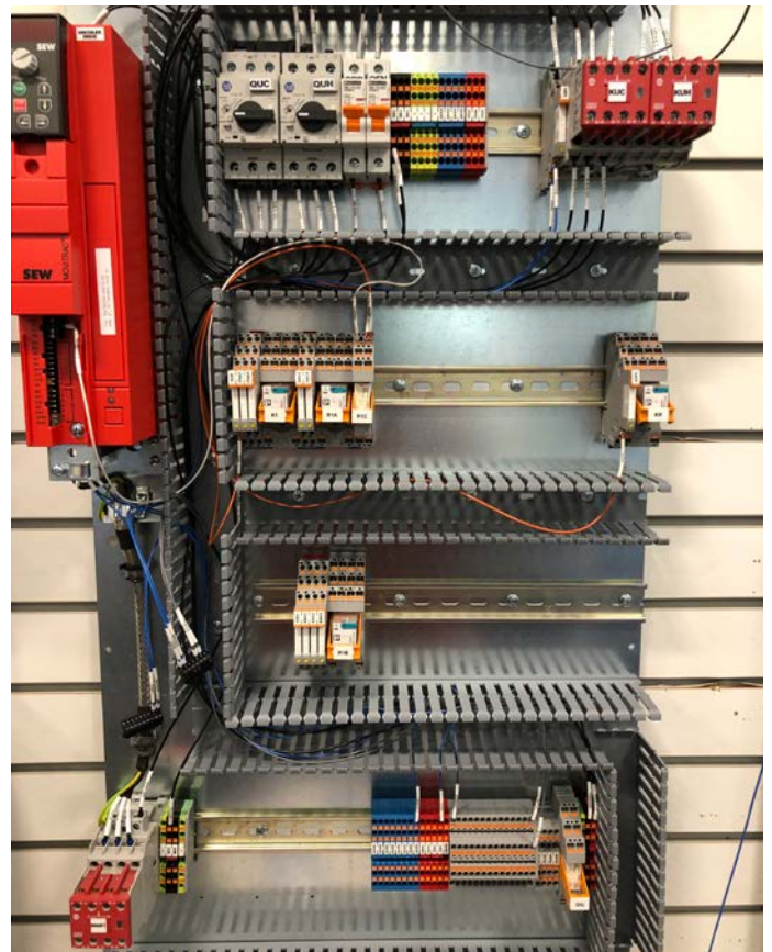
Figure 3: Phoenix Contact assists with rail assembly.
