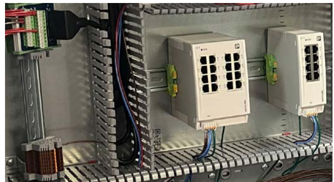
Figure 3: The FL 2000 Ethernet managed switches were more cost-competitive and improved the network reliability.
