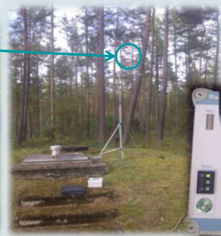
Water supply well 868 MHz (Slave) 9,6 kbps 8 dBi Yagi
