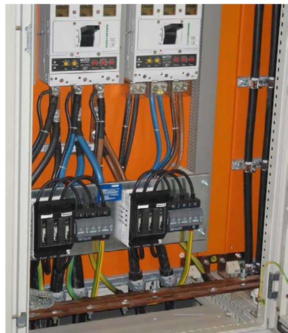
Figure 11: 100,000 A SPD for use at power line input feeds
