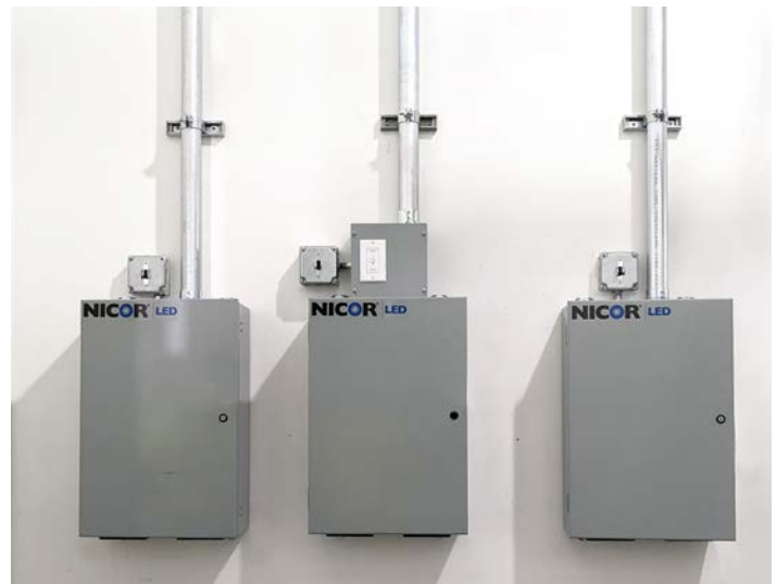
Figure 3: The IMS is certified to UL 2108 as a Low Voltage Lighting System.
