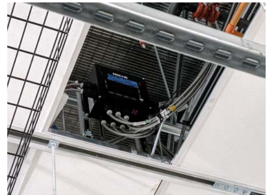
Figure 1: Distribution boxes have color-coded, uniquely keyed components for error-free connectivity.
