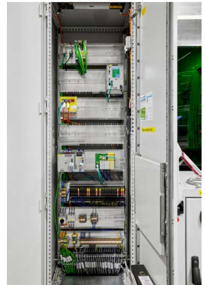
Figure 3: In addition to functionally safe system automation, the RFC 4072S PLCnext Control provides comprehensive diagnostics.
