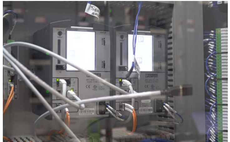
Figure 2: The redundant RFC 460R controllers are connected on a plant-wide fiber-optic ring. The controllers employ PROFINET Media Redundancy Protocol (MRP) to provide fault recovery time in milliseconds, providing the highest level of resilience for control and communications.
