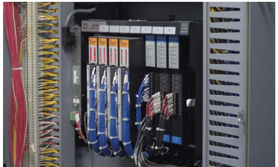
Figure 1: The old PLC, installed in the 1990s, was in danger of failure, which could have disastrous consequences for the residents who rely on the water supply.
