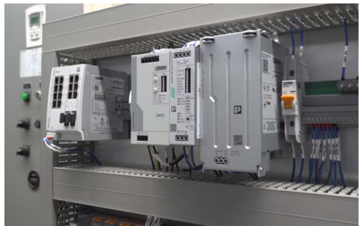
Figure 3: Each station on the ring has a DC UPS battery backup for power redundancy. This further increases the system’s reliability and resilience.
