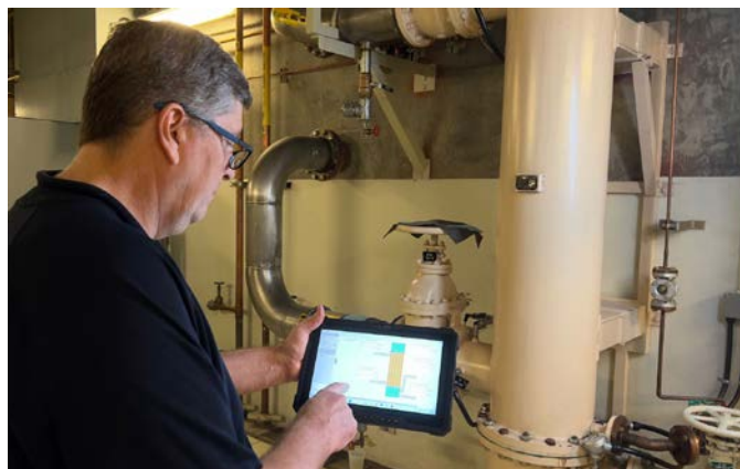
Figure 3: The technicians now have access to real-time SCADA data right on the plant floor, so they can take action on alarm situations much more quickly.
