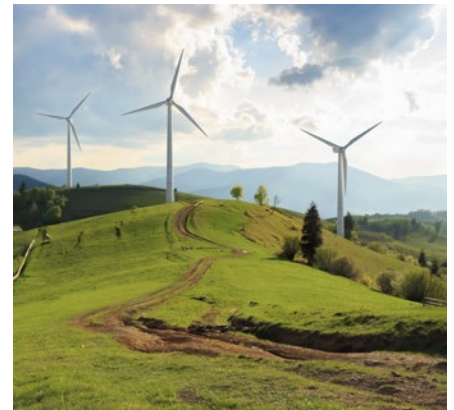
Protected signal circuits at lofty heights
