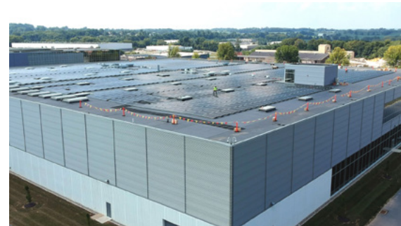
Solar panels generate nearly 1 MW of electricity at Phoenix Contact USA headquarters
