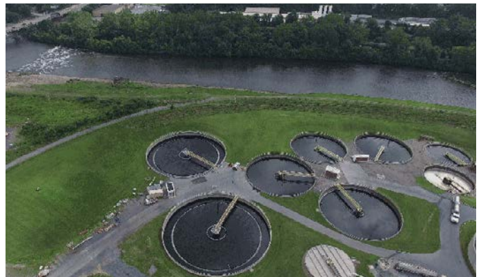
The Lehigh County Authority's main wastewater treatment plant – nearly a century old – needed an upgraded SCADA system to accommodate increasing demands.
