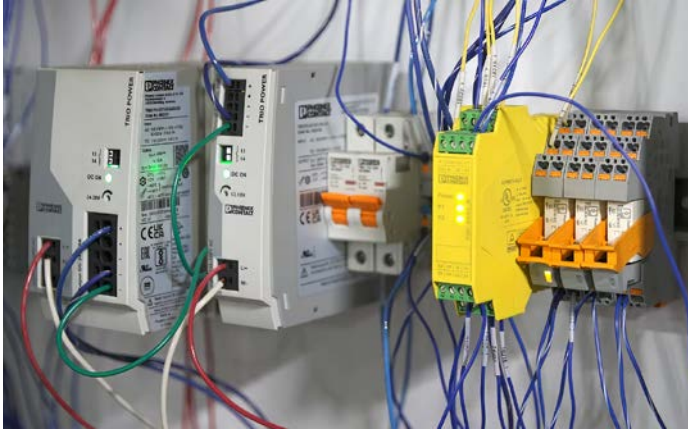
Figure 3: NJ Tool Repair trusts a variety of Phoenix Contact products, including power supplies, surge suppressors, safety relays, and more. Phoenix Contact’s Limited Lifetime Warranty was very appealing.
