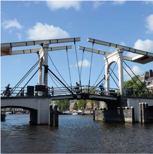
Drawbridge used for road traffic
