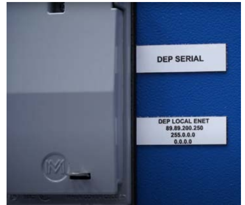
Figure 3: NSRW uses the NEO to print different types of labels, making it easy to identify terminal blocks, IP addresses, device functionality, and more.
