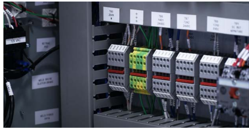
Figure 4: NSRW uses a variety of Phoenix Contact terminal blocks and fuse holders, including the QUATTRO series.
